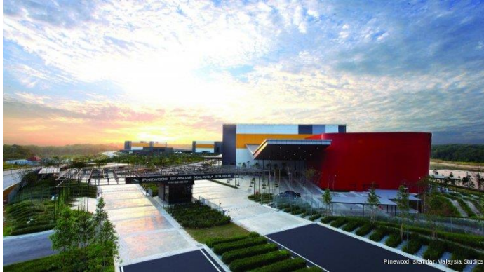
Image 3: Pinewood Iskandar Malaysia Studios Complex, a building with green facilities (Pinewood Malaysia Studios, n.d.).
